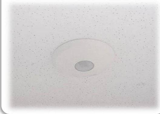
Motion Sensor for Restroom Lighting Control
