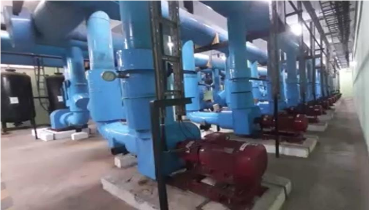
Existing System: Primary and secondary pump system
